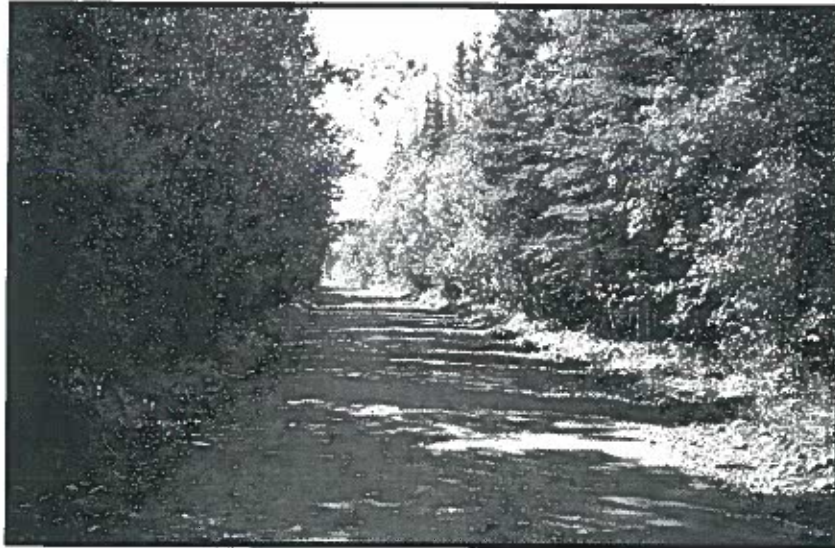
The narrow road will require widening to provide space for two vehicles to pass.
