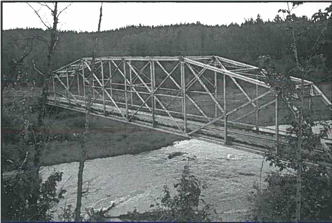
The one-lane Lakina River bridge was originally erected over either the Tonsina or Klutina Rivers, and relocated to its present location at Milepost 44 in 1981.
