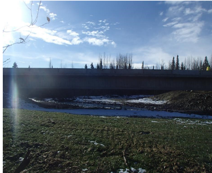
Figure 6-9. Chokosna River Bridge (BR 1193), Upstream Looking Downstream
