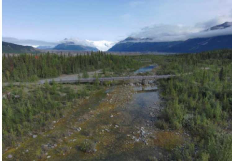
Figure 6-36. Kennicott River Bridge (BR 6005), Downstream Looking Upstream
