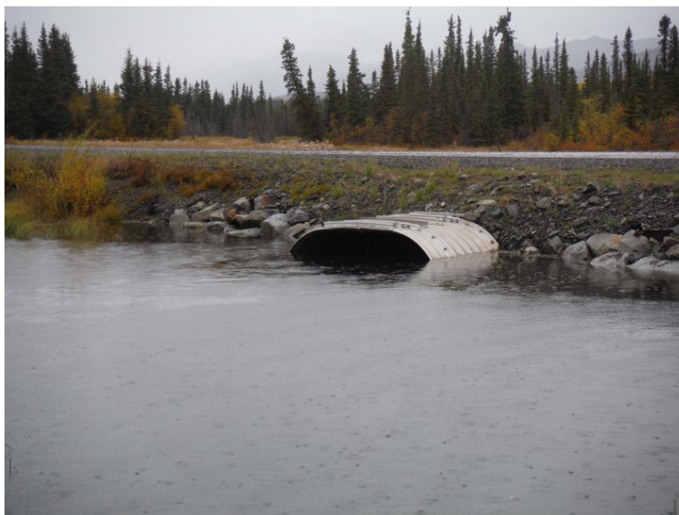
Figure 6-8. Chokosna River Tributary (MC 15) Cross Culvert, Upstream Looking Downstream
