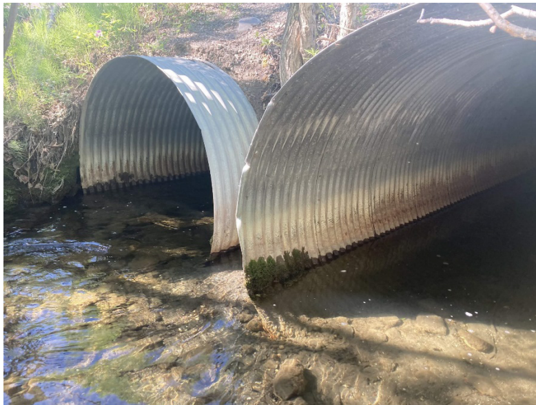
Figure 6-26. Long Lake Creek Cross Culvert (MC 8), Downstream Looking Upstream
