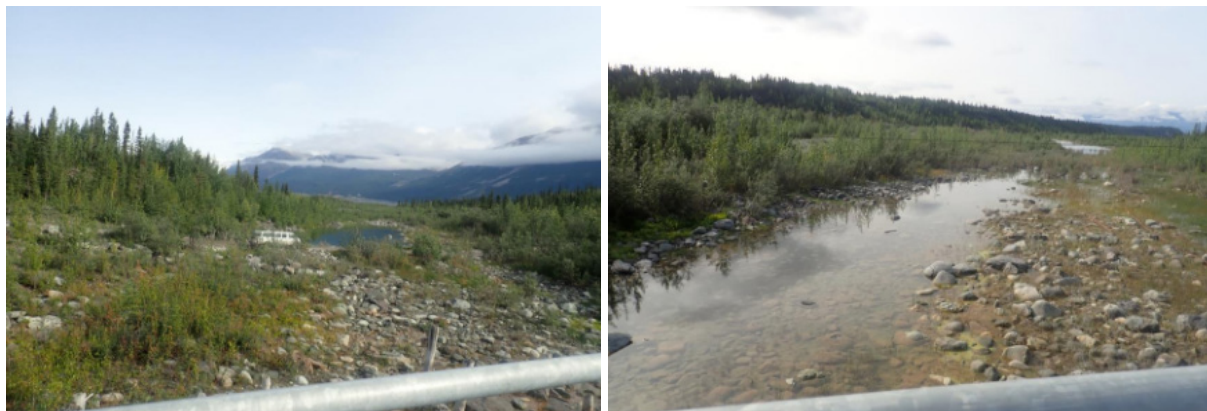
Figure 6-37. Kennicott River Bridge (BR 6005), Looking Upstream and Looking Downstream
