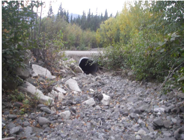
Figure 6-19. Ruth Creek Cross Culvert (MC 10), Upstream Looking Downstream
