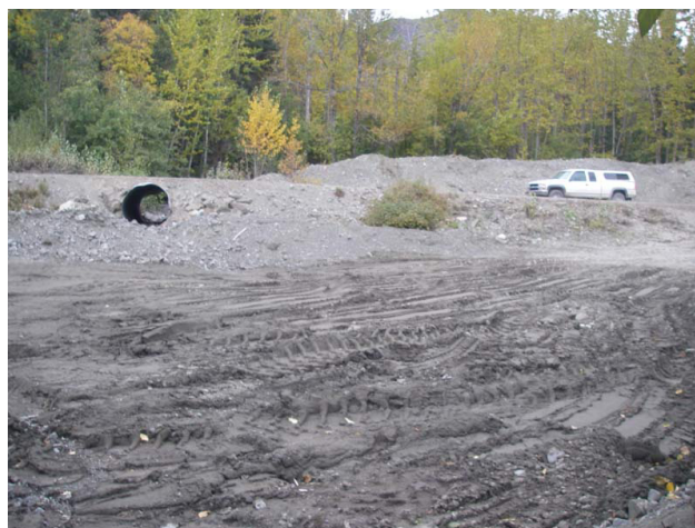
Figure 6-20. Ruth Creek Cross Culvert (MC 10), Downstream Looking Upstream
