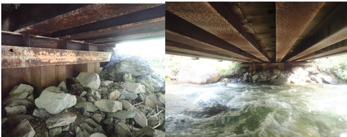
Figure 6-18. Gilahina River Bridge (BR 1194), Looking Upstream, at Left and Right Abutment
