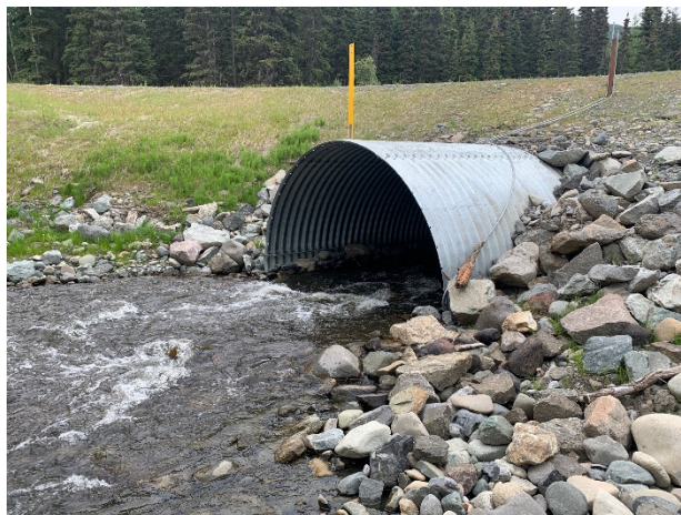
Figure 6-22. Crystal Creek (MC 9), Looking Upstream (post-improvement project)
