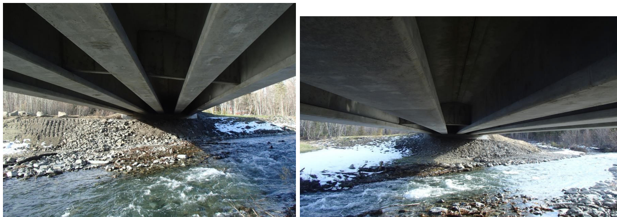
Figure 6-10. Chokosna River Bridge (BR 1193), Looking Upstream, Right and Left Abutment
