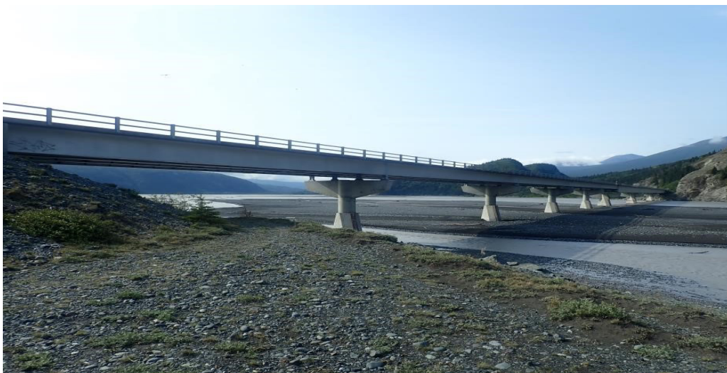
Figure 6-2. Copper River (Chitina) Bridge (BR 0205), Upstream Looking Downstream
