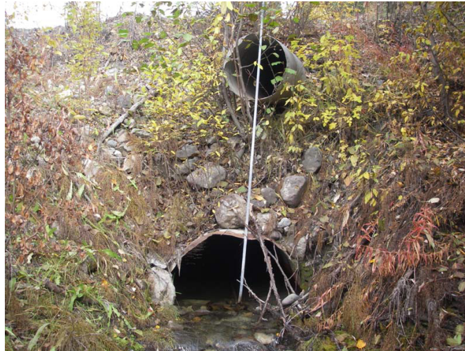
Figure 6-29. Tractor Creek Cross Culvert (MC 3), Downstream Looking Upstream
