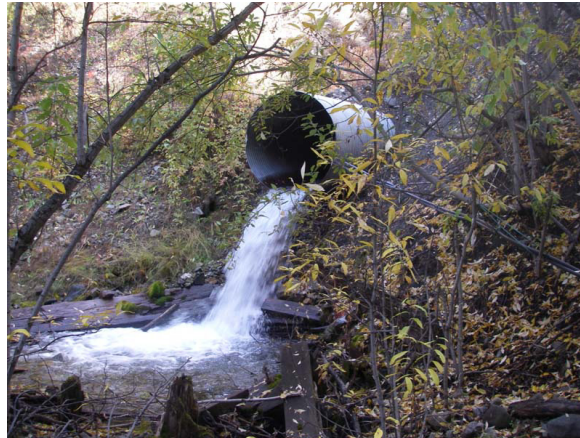
Figure 6-31. Swift Creek Crossing (MC 2), Downstream Looking Upstream
