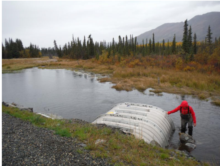
Figure 6-7. Chokosna River Tributary (MC 15) Cross Culvert, Upstream Side Looking South
