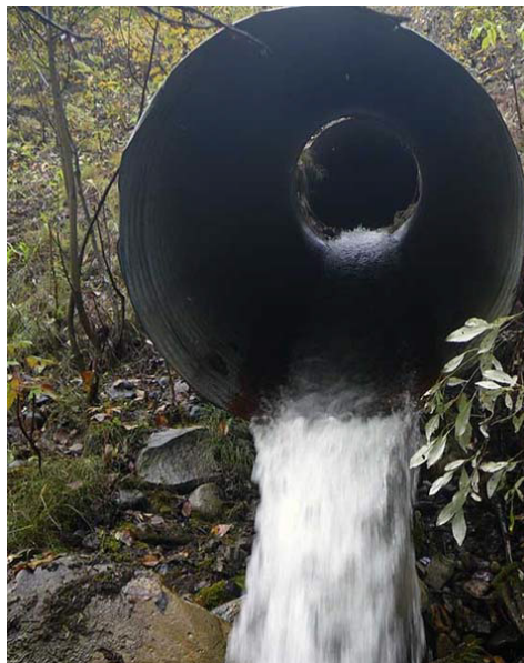
Figure 6-34. Farm Creek Cross Culvert (MC 1), Downstream Looking Upstream
