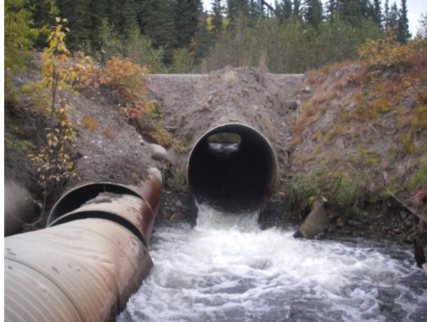
Figure 6-21. Crystal Creek (MC 9), Downstream Looking Upstream (pre-improvement project)
