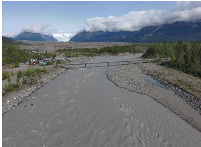
Figure 6-35. Kennicott River Bridge (BR 6004), Downstream Looking Upstream
