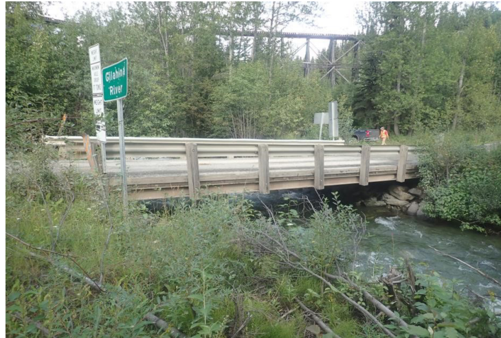
Figure 6-17. Gilahina River Bridge (BR 1194), Downstream Looking Upstream
