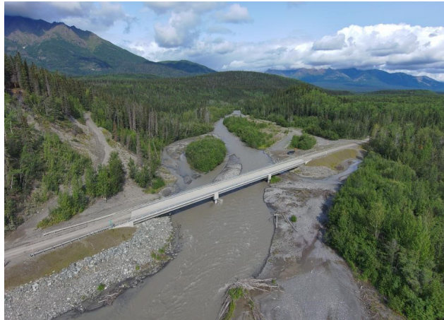
Figure 6-23. Lakina River Bridge (BR 1195), Upstream Looking Downstream
