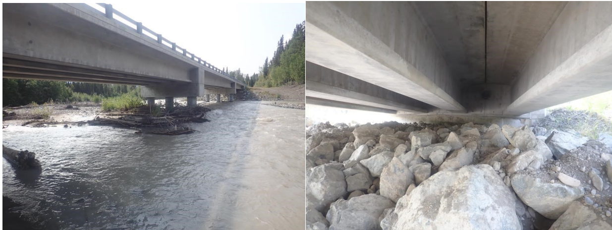
Figure 6-24. Lakina River Bridge (BR 1195), Looking Upstream, Piers and Right Abutment
