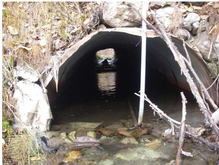
Figure 6-30. Tractor Creek Cross Culvert (MC 3), Upstream Looking Downstream
