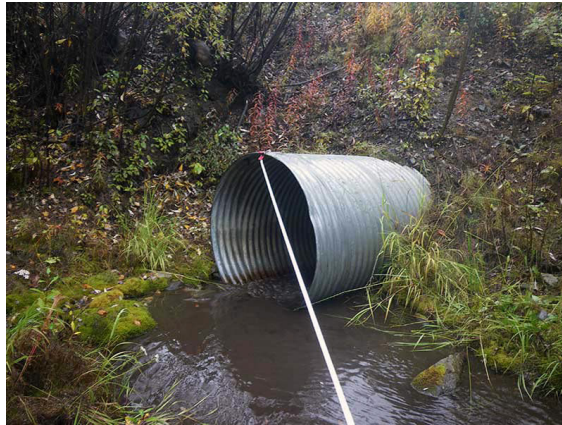
Figure 6-33. Farm Creek Cross Culvert (MC 1), Upstream Looking Downstream
