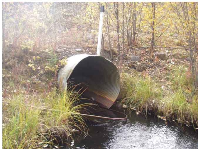
Figure 6-28. Long Lake Creek Crossing (MC 7), Downstream Looking Upstream
