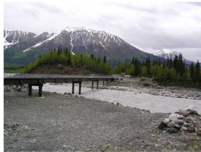
Kennicott River bridge crossing
