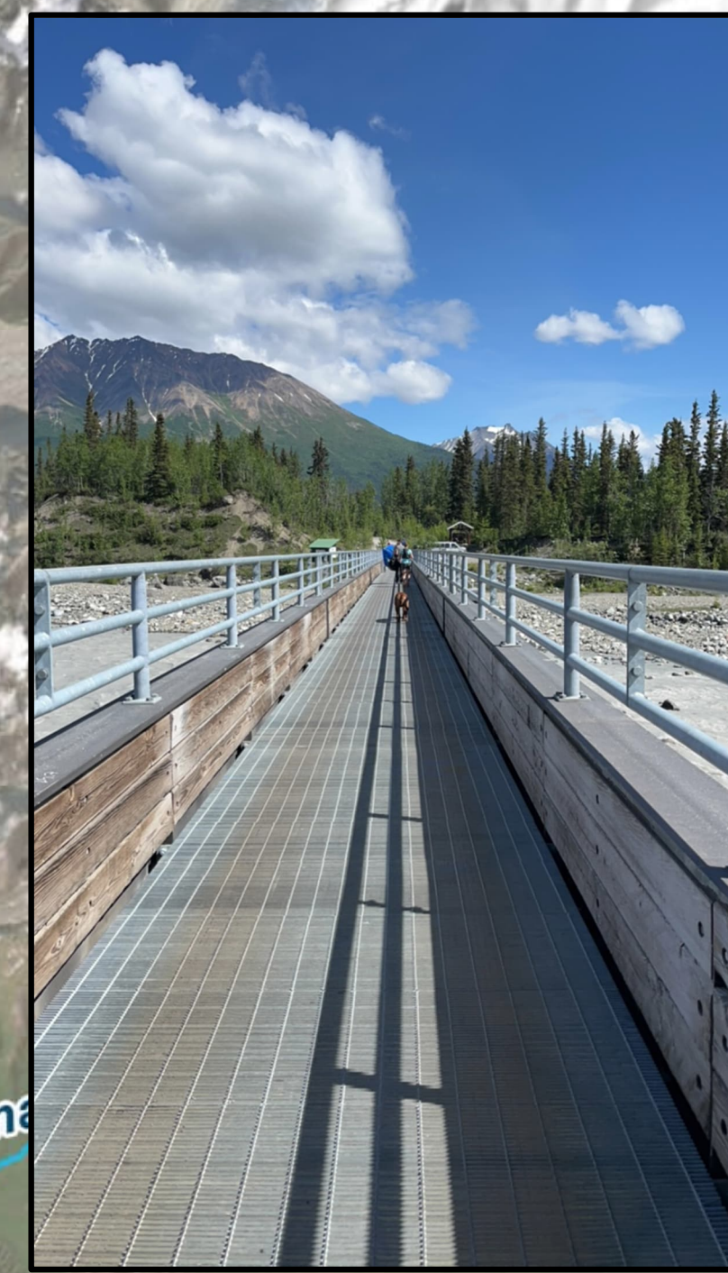
Kennicott River Bridge Crossing Improvements
